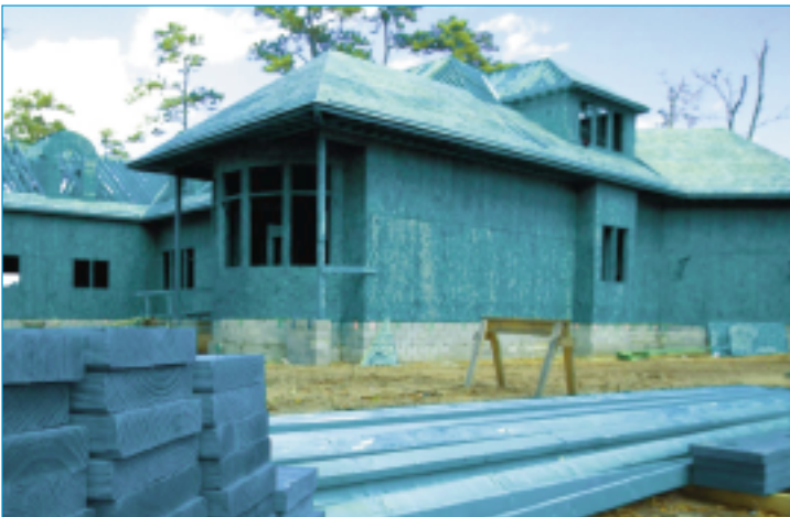
Wood components treated in the two-step process are considered non-hazardous, non-polluting, and non-carcinogenic per the limits of FIFRA, making them safe to use throughout a home.
