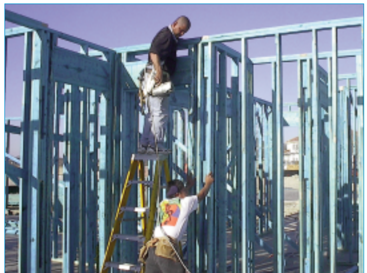
Wood that has been treated in the two-step process does not require any special handling. These components can be sawed, mechanically anchored, adhered, and painted just the same as untreated wood components.
